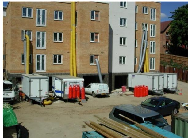
These systems are the most efficient trailer drying systems available and can cost effectively do the work of over 50 traditional dehumidifiers from just one 110v or 230v socket and at reduced environmental impact.
